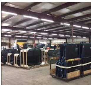
Burnsville Warehouse – LM Clip Only Screwed to the Beam
