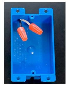
Remove wall switch cover. Remove switch and cap wires
