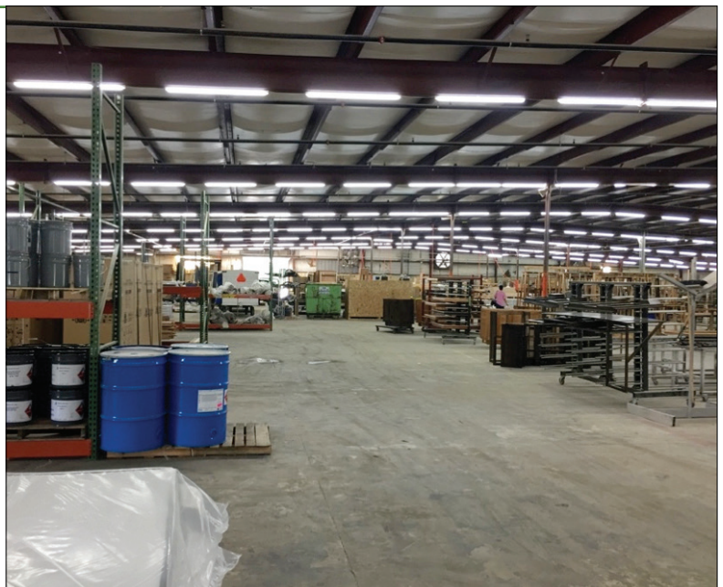
42 Foot Candles Purlin Mounted LMK422 Sticks
