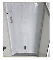
Remove lamps and if required by local code or utility rebate program, the ballast. No need to remove the lamp holders.
